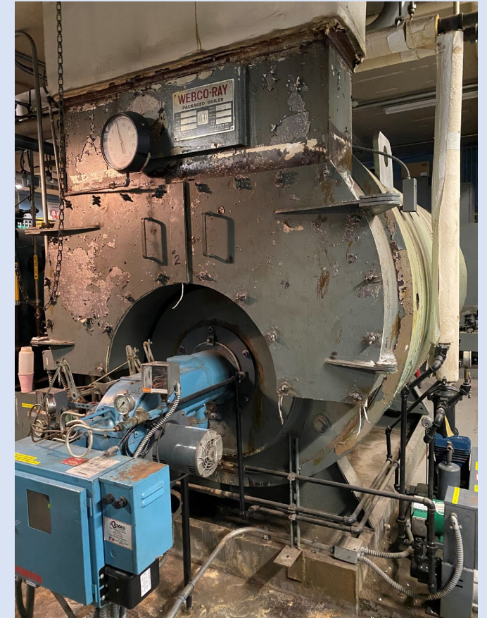
Boiler at Judy Jacobs Parkway installed in 1959
